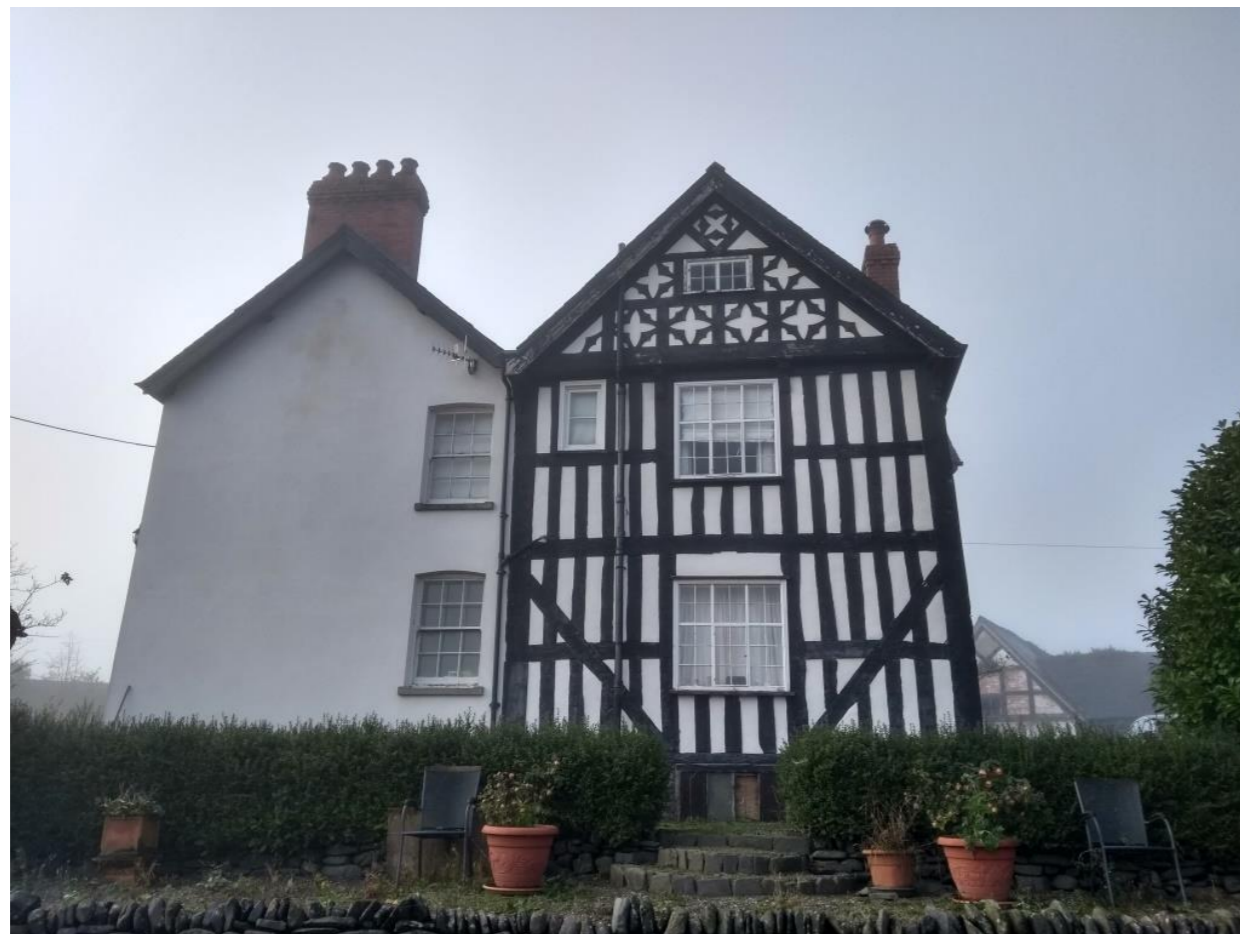
Image 12.19: Perth Eiryn listed building east face showing fine timber-frame construction
